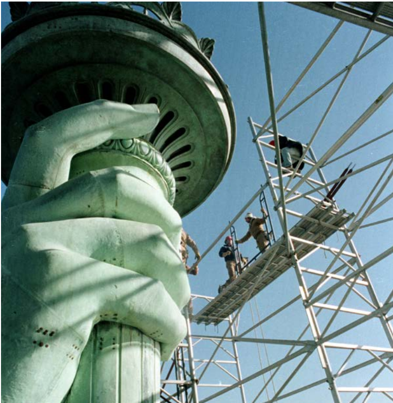
Workers fix the torch in 1985.
